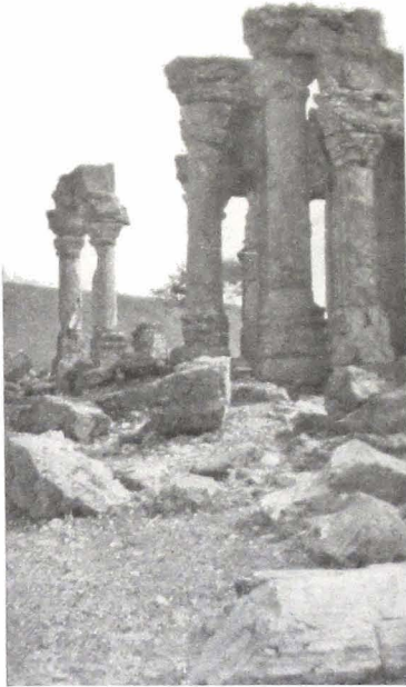
TEMPLES UNMISTAKABLY GREEK How the Hellenic Spirit Drifted to the Vale of Kashmir Is a Lost Legend
